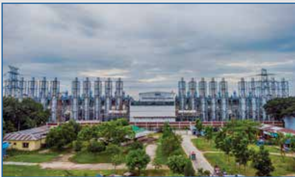
United Ashuganj Energy Limited - 195 MW Gas fired IPP Plant at Ashuganj, Brahmanbaria
