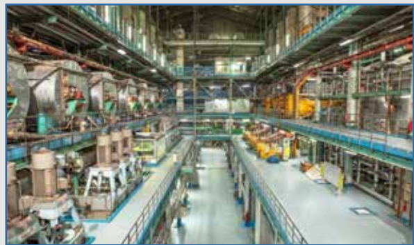
City Sugar Industries Limited - a Sugar Refinery at Rupganj, Narayanganj
