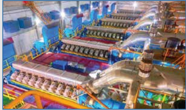
KSRM Power Plant Limited – 55.80 MW LNG fired Captive Power Plant at Kumira, Chattogram
