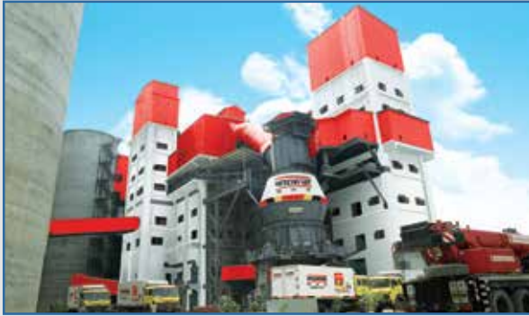
Bashundhara Industrial Complex Limited - Cement Manufacturing plant at Mongla Port I/A, Mongla, Bagerhat, Khulna.
