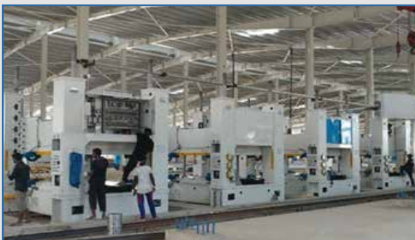
Butterfly Manufacturing Company Limited - A Refrigerator Manufacturing Plant [Under Implementation]
