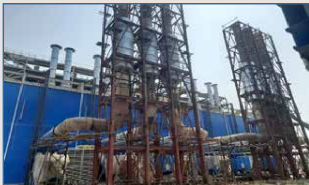
KSRM Power Plant Limited - 55.80 MW Power Plant at Kumira, Chattogram
