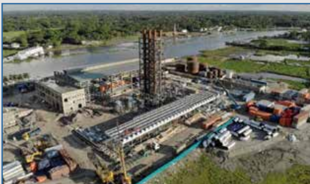
Chandpur Power Generations Limited - a 115 MW HFO fired IPP Power Plant at Chandpur [Under Implementation]
