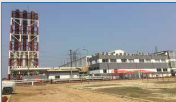
Karnaphuli Power Limited - a 115 MW Power Plant at Potiya, Chattogram
