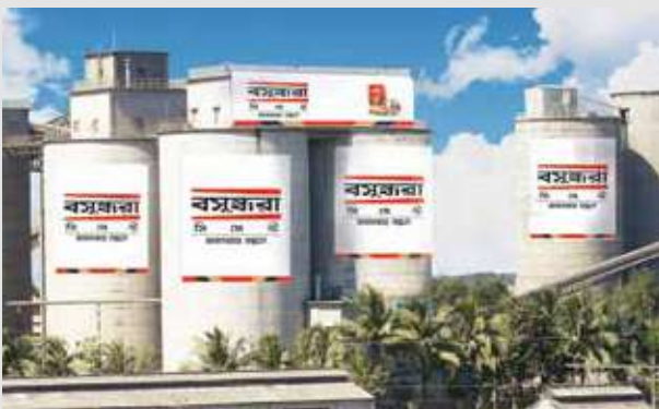
Bashundhara Industrial Complex Limited - A cement manufacturing mill at Mongla, Bagerhat
