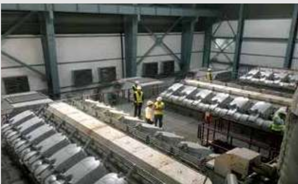
Zodiac Power Chittagong Limited - a 54.363 MW HFO fired IPP Power Plant
