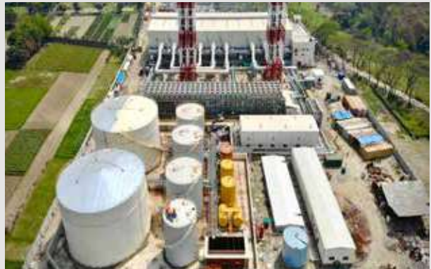
Manikganj Power Generations Limited - a 162 MW HFO fired IPP Power Plant [Under Implementation]
