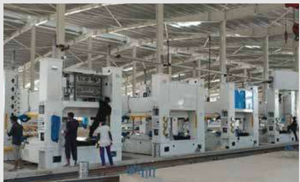
Butterfly Manufacturing Company Limited - A Refrigerator Manufacturing Plant [Under Implementation]
