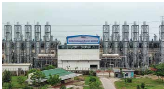
United Ashuganj Power Limited
