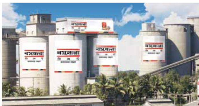
Bashundhara Industrial Complex Limited (A cement manufacturing mill at Mongla, Bagerhat)
