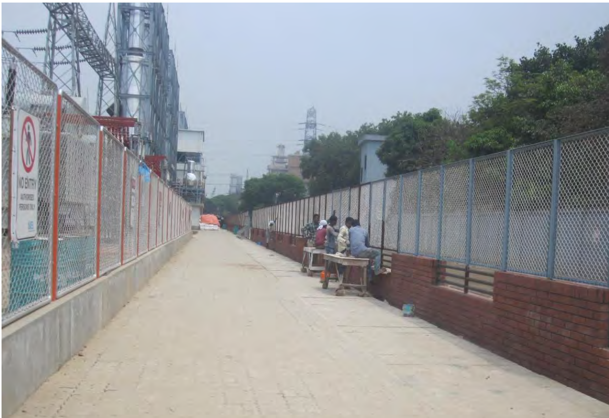
Figure 6-1: Paved View of the Plant Premises
